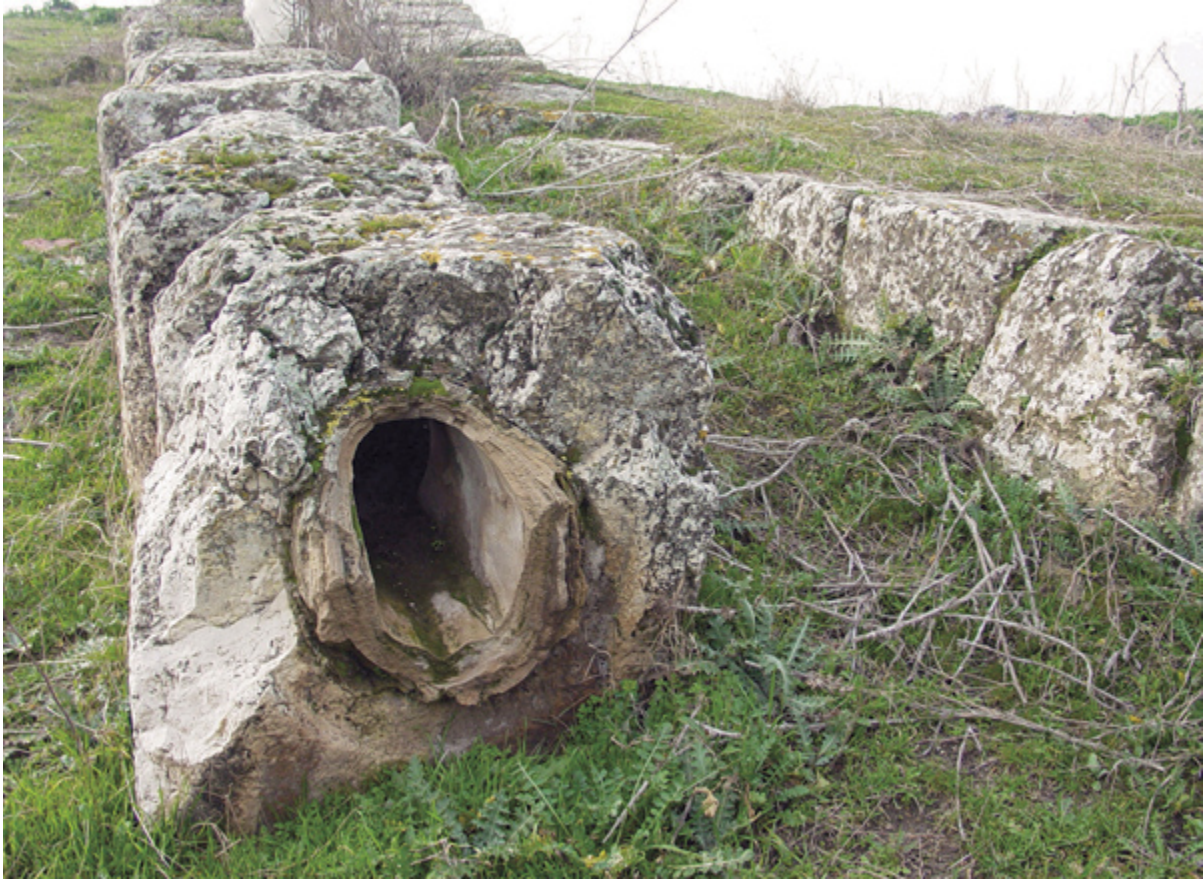
Laodicea: calcified siphon that once brought water into the city (Rev 3:15-16)
