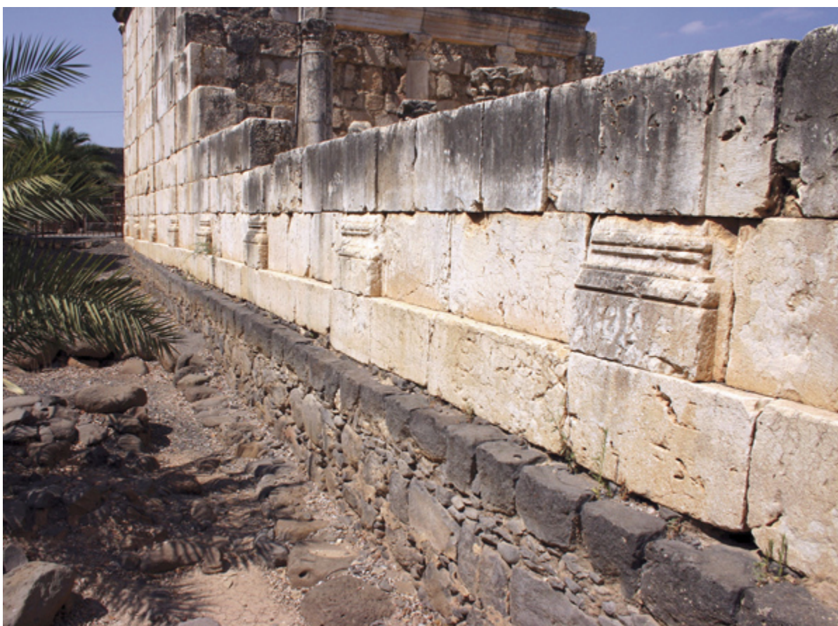
Black basalt foundation wall of an earlier synagogue upon which the rebuilt limestone walls of the sixth-century synagogue at Capernaum are visible.
