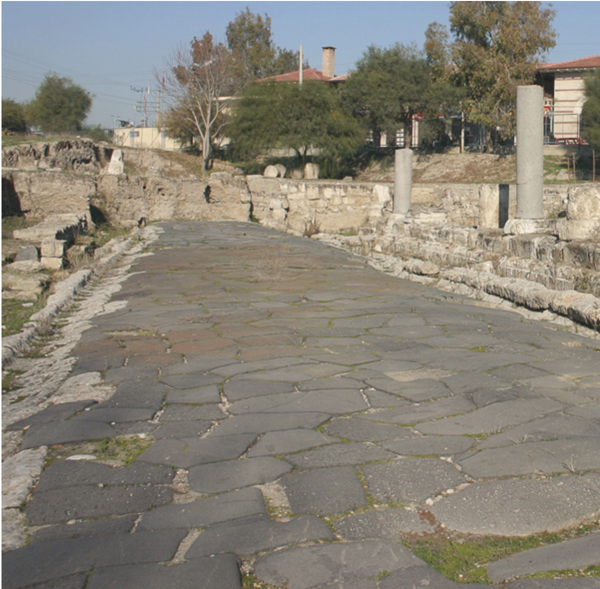
Tarsus: one of the main streets from the days of Paul. Note the basalt paving stones, the white limestone curbing, and the remains of buildings that line the right side of the street.
