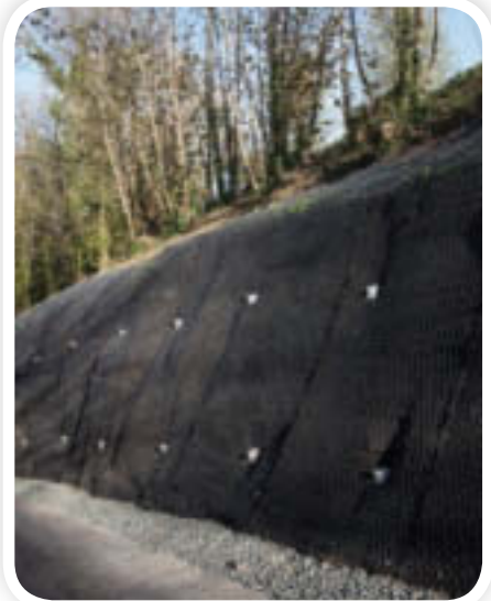
One way to avoid having a house collapse as the hillside is eroded is to lay down plastic that minimizes erosion.
