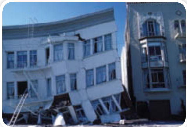
When a powerful earthquake struck the San Francisco area in October 1989, much of the worst damage occurred in areas such as the Marina District, which was built on loose soil.
